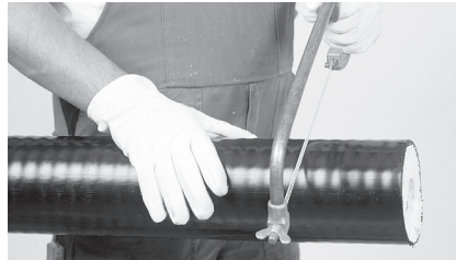
2 Cut the casing pipe with saw.
