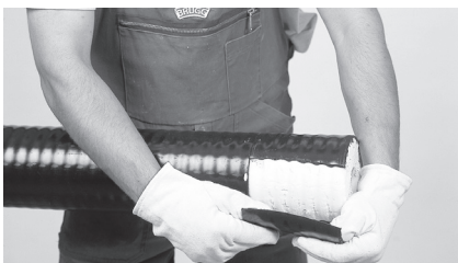
4 Peel off the casing.
